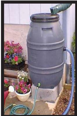
A recycled, food-grade barrel washed, refitted and ready to collect rain.
