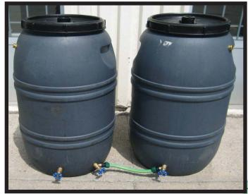
Barrels connected at the bottom
